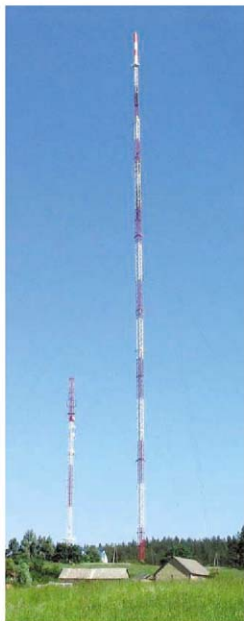
The advantages of height. Atmospheric measurements are made on the tall tower (300 m). The tower, located near Białystok in eastern Poland, is part of the CarboEurope tall tower network. Similar networks exist in North America and more sparsely in other parts of the world.
